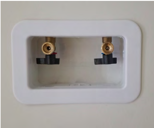
Laundry Machine shut-off valves. Typically located beside or behind laundry machine. Refer to Homeowners Manual for suggested shut off times.
